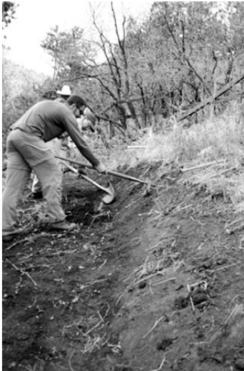
Backslope work on a trail.
