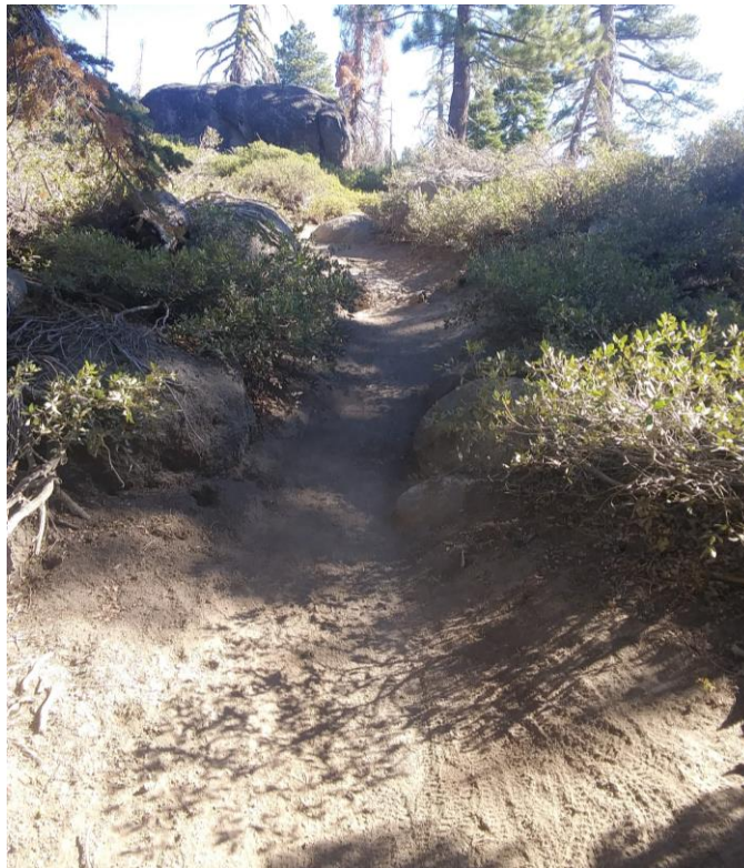
Numerous steep sections are eroding and becoming braided, such as these sections at 18% (above) and 25% (below).
