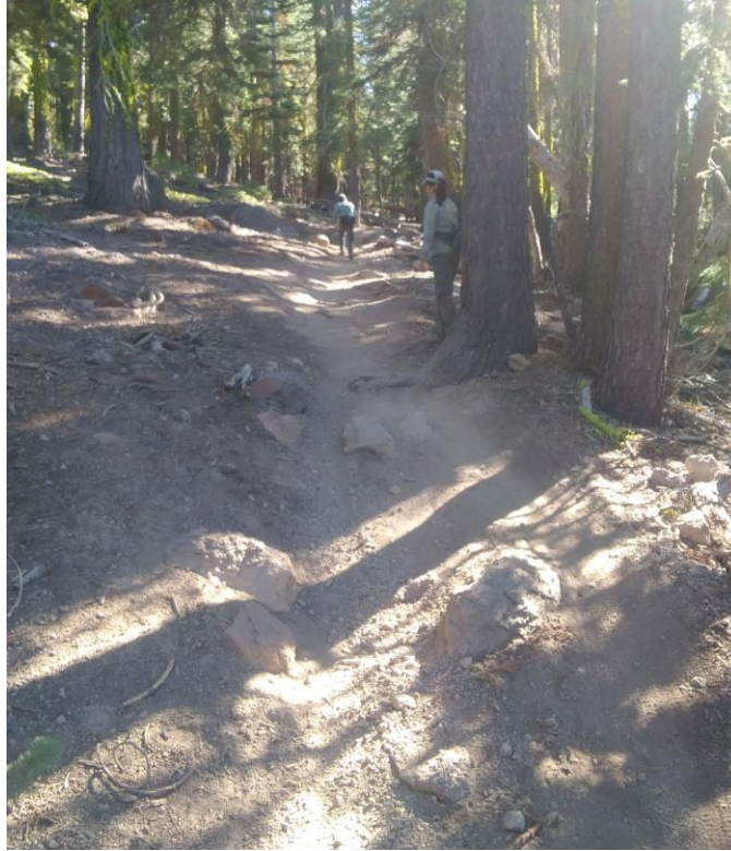
Numerous steep sections are eroding and becoming braided, such as these sections at 18% (above) and 25% (below).
