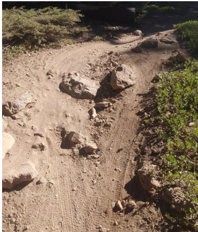
Poorly routed, steep trail is causing braiding.
